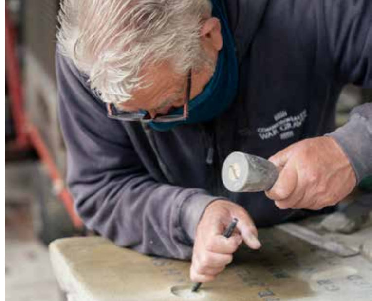
Stone repairs Cliveden War Cemetery, UK
